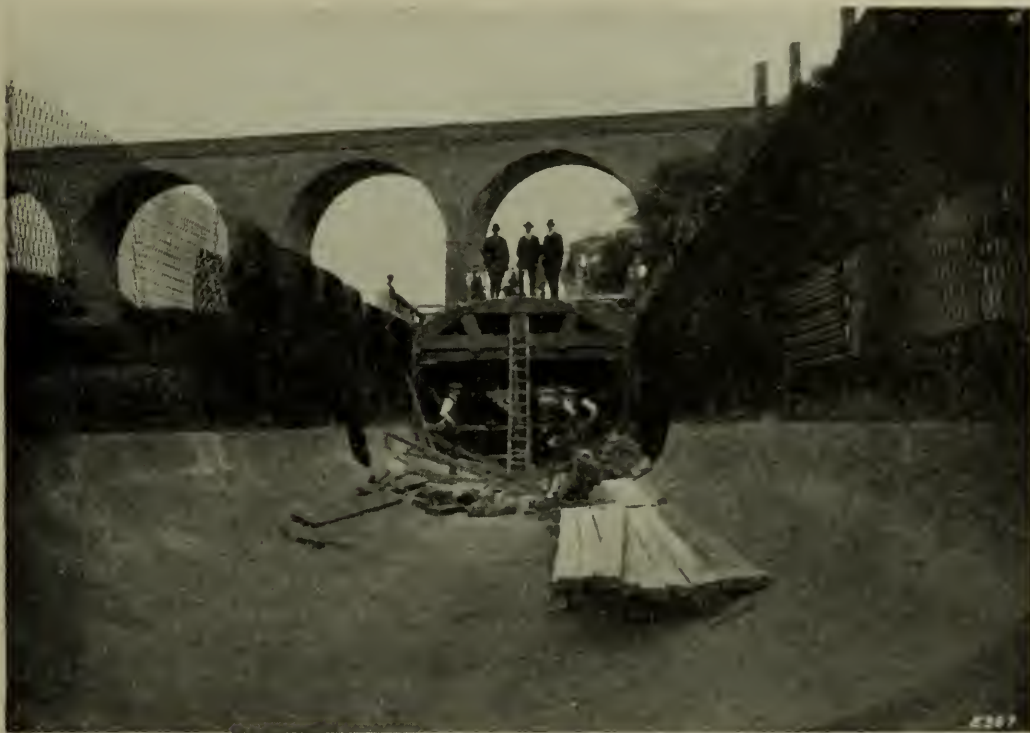
CRIMDON DENE CULVERT—LOOKING EAST.
